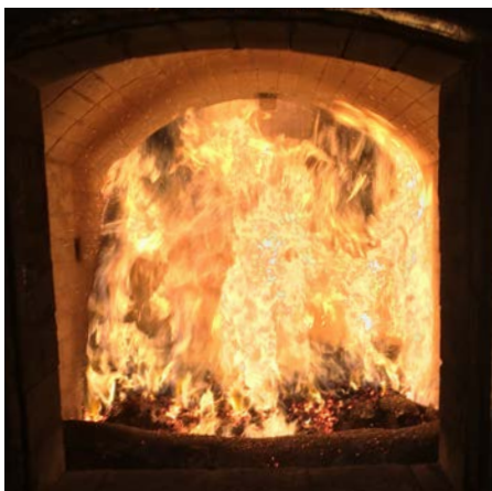
KPR System 5 MW
